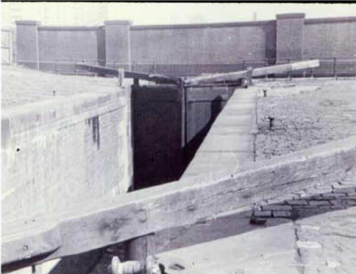
Lock 5 Head Gates - view towards Oldfield Road
