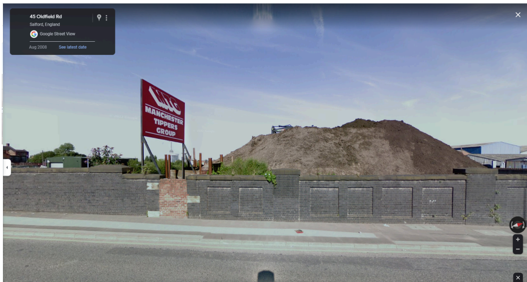
Google streetview from 2008 showing original access to the towpath, now bricked up.
