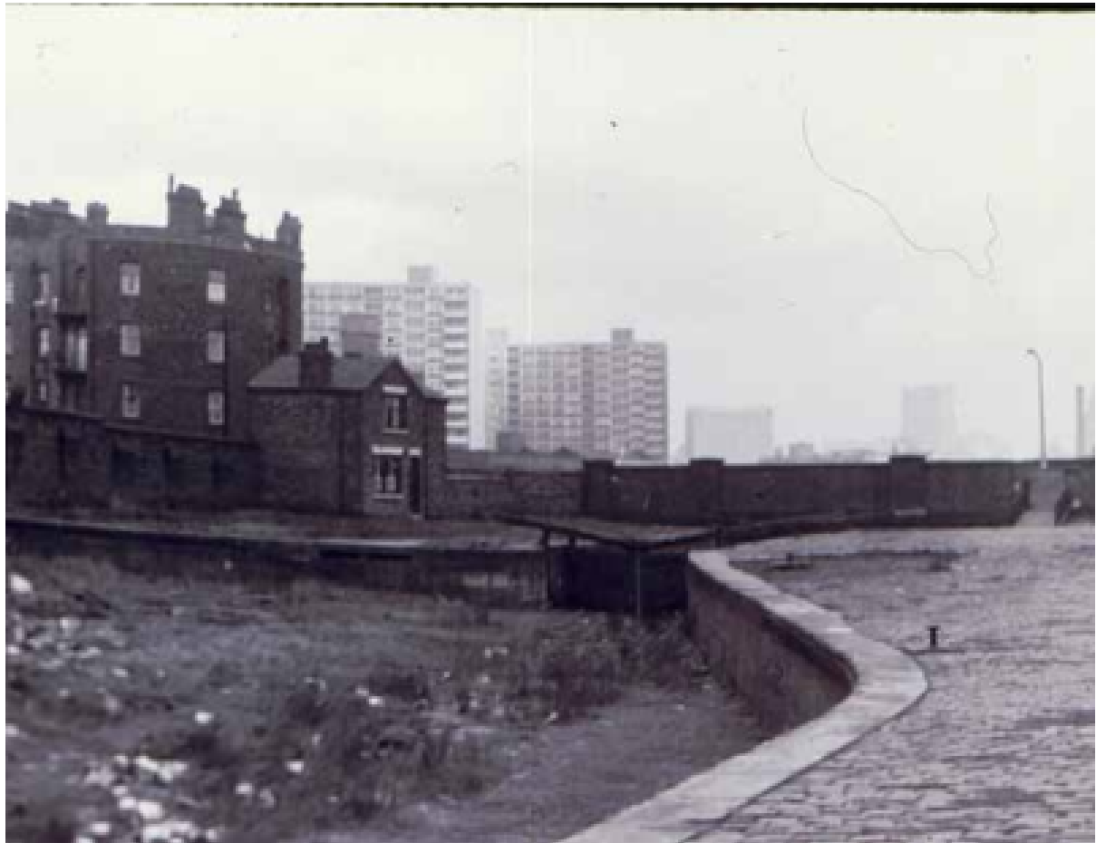
View of Lock 5 looking towards the Oldfield Road parapet with Oldfield Dwellings to the left. Source: H2O Urban's Design and Access Statement.
