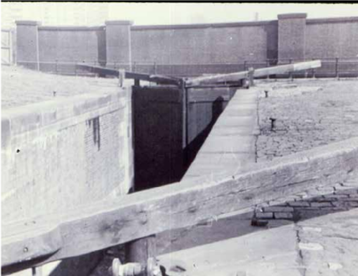
Lock 5 Head Gates - view towards Oldfield Road
